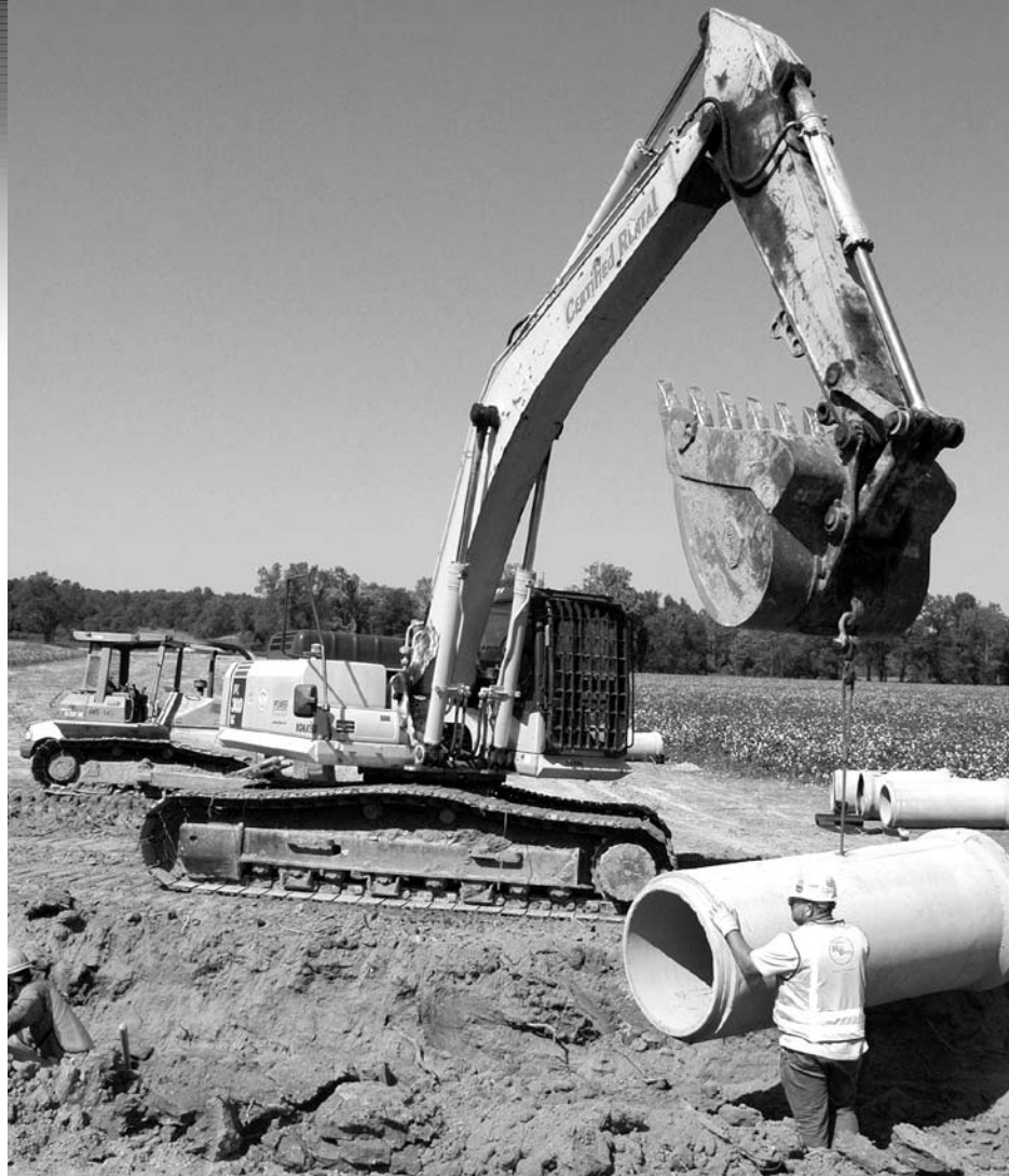
A Hill Bros. operator uses a Komatsu PC300LC-7 excavator to set pipe on a highway project near Memphis. The company, which owns a vast number of Komatsu machines, used a D65 dozer for backfilling operations.
