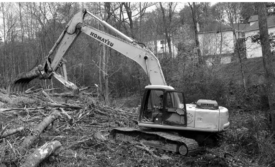
Farris Excavating uses this Komatsu PC200-6 with a grapple rake and thumb attachment to clear trees for a residential subdivision on the west side of Knoxville.
