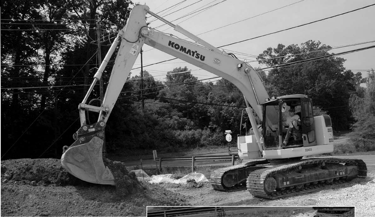
A Marvin Sledge Construction operator uses the Komatsu PC228USLC excavator to put in 18-inch pipe for a sewer upgrade in Knoxville, Tenn.
