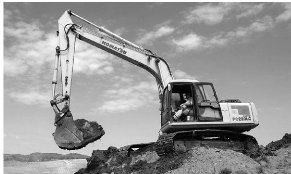
A Smith Excavating operator moves dirt with a Komatsu PC220LC excavator.
