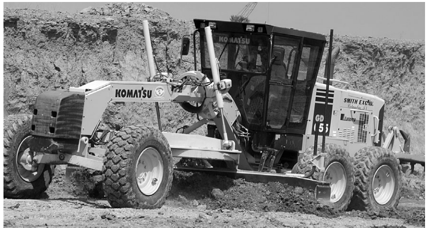
Included in Smith Excavating's Komatsu fleet is this GD655, used here for grading on a jobsite near Columbia.
