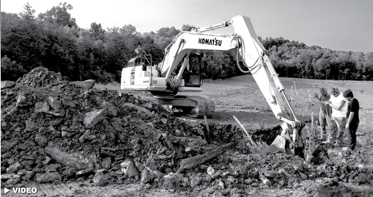
Using a Komatsu PC240LC excavator this Underground Pipe & Construction operator digs around a water line on a residential project in Nashville. “We started with Komatsu,” said Co-owner Ricky Williams. “They are great machines that last.”
