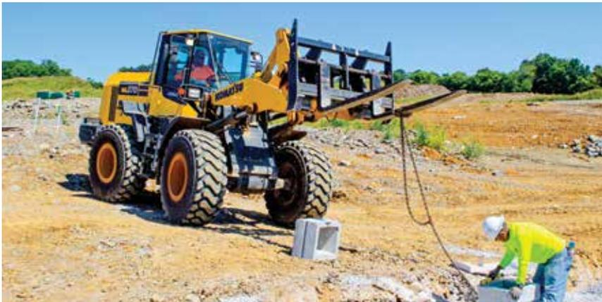
An operator uses one of Covenant Constructors' Komatsu WA270 wheel loaders to help set a concrete form.
