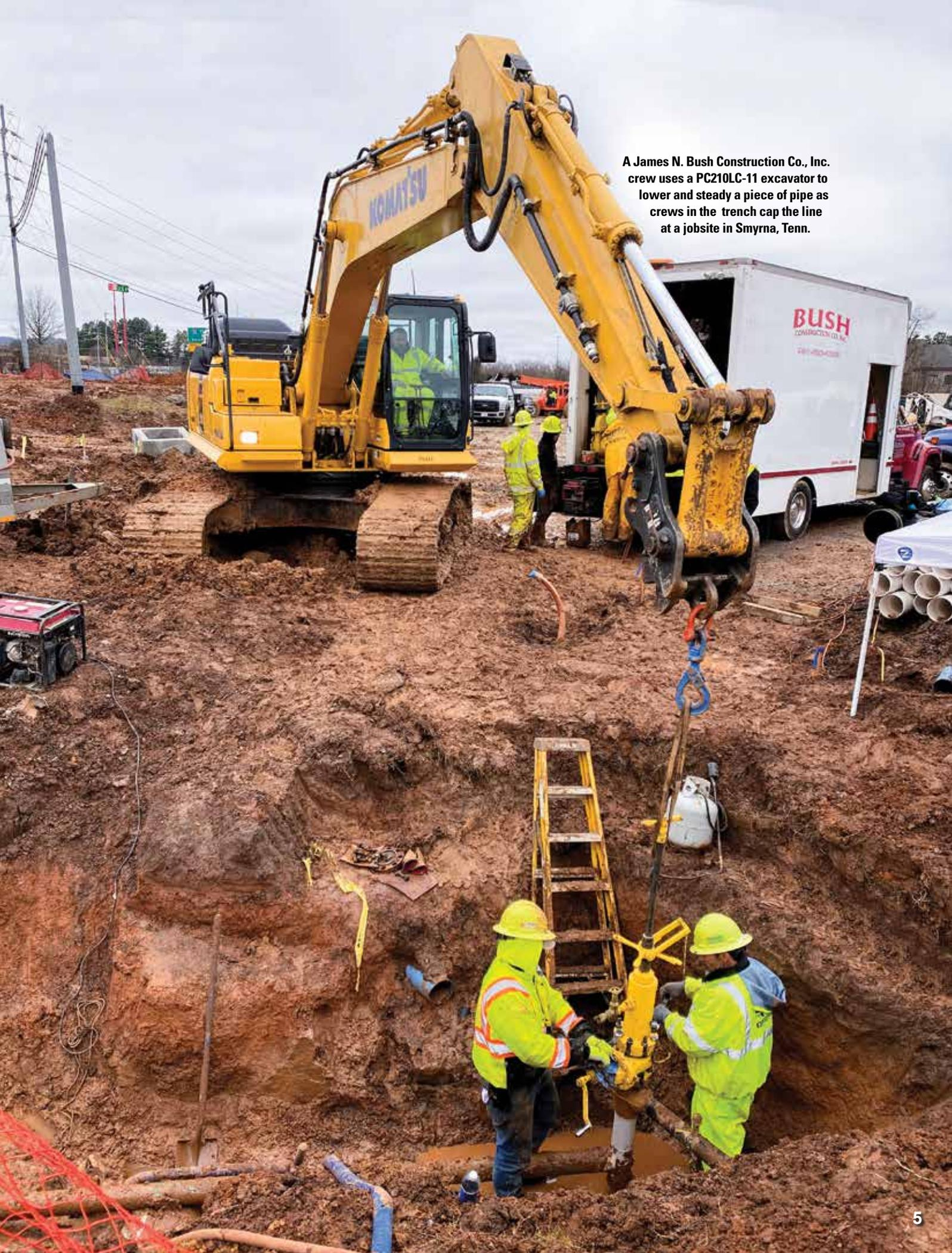
**A James N. Bush Construction Co., Inc. crew uses a PC210LC-11 excavator to lower and steady a piece of pipe as crews in the trench cap the line at a jobsite in Smyrna, Tenn.**
