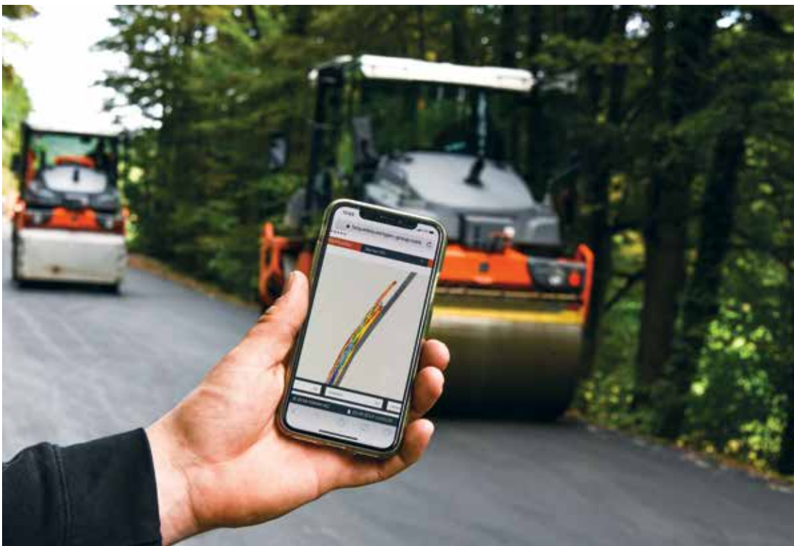
HAMM's new WITOS HCQ system records and displays all data gathered by connected HAMM rollers during the compaction process, providing real-time analysis from any location.
