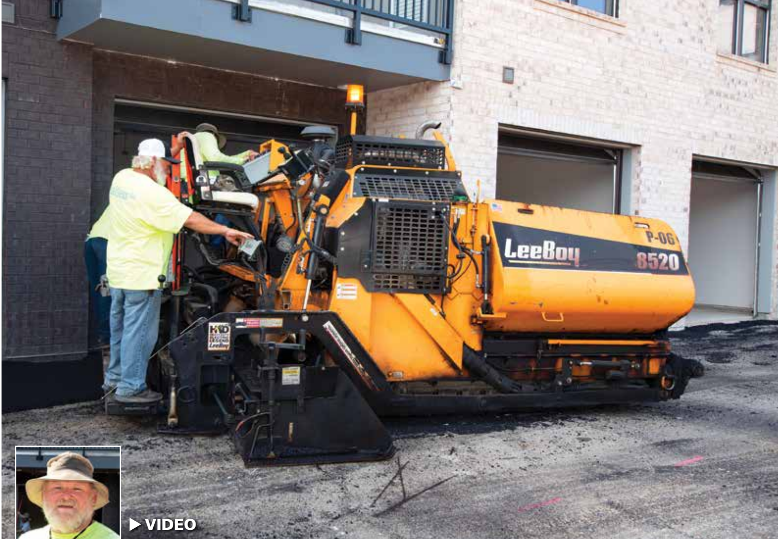
At the Apartment One complex in Chattanooga, Tenn., Phaltless Inc. Foreman Dennis Bales operates a LeeBoy 8250 compact paver as he lays down the final layer of asphalt.
