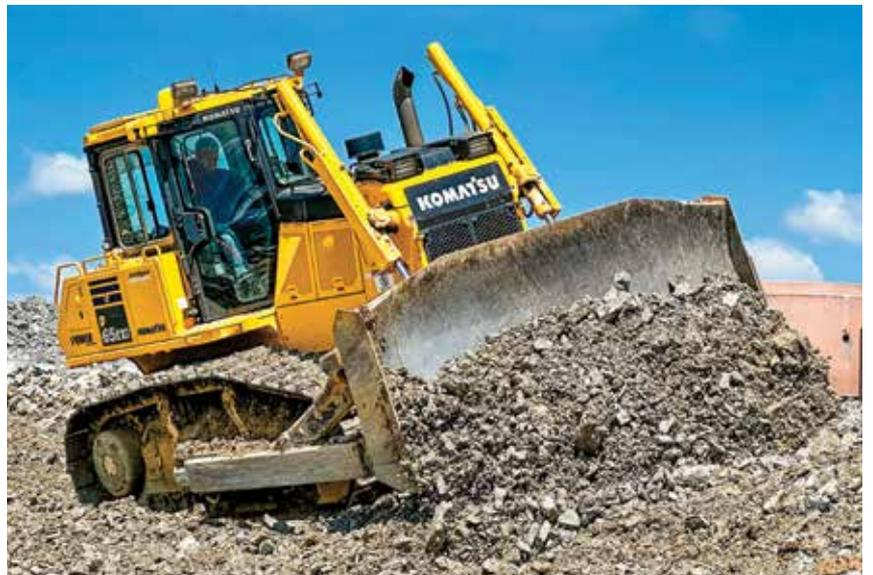
With a Komatsu D65EXi IMC 2.0 dozer, an operator fine grades a slope.
