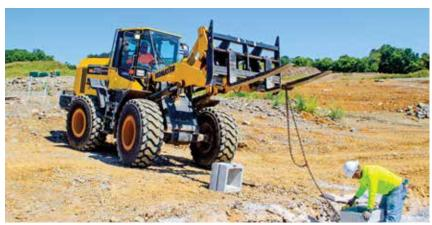
An operator uses one of Covenant Constructors' Komatsu WA270 wheel loaders to help set a concrete form.
