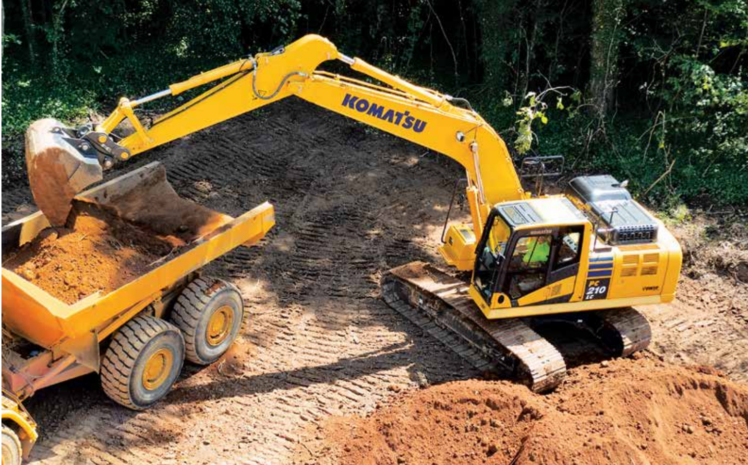
An operator uses a Komatsu PC210LC excavator to load material into a haul truck at the Highland Ridge subdivision in Knoxville, Tenn.
