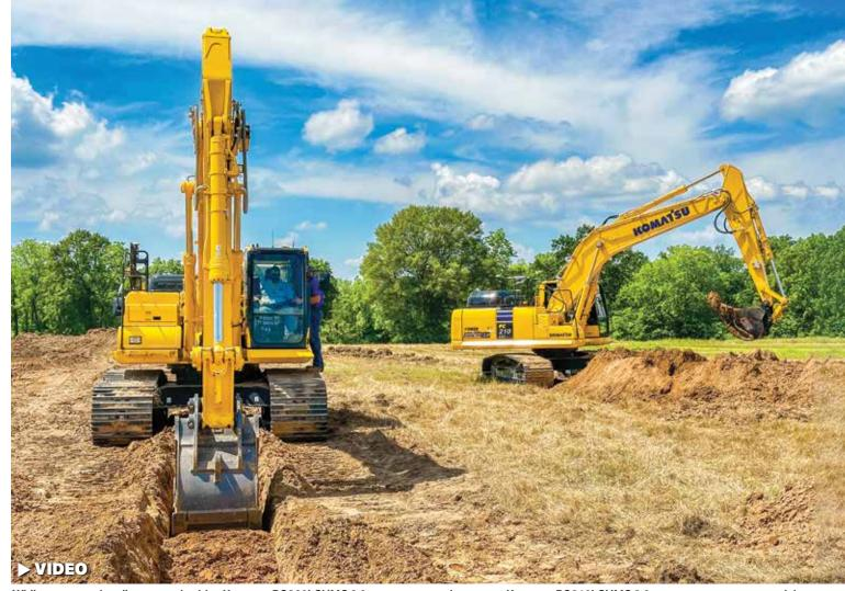
While one attendee digs a trench with a Komatsu PC360LCi IMC 2.0 excavator, another uses a Komatsu PC210LCi IMC 2.0 excavator to move material.
