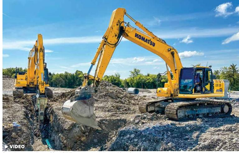
Surrey Homes uses a Komatsu PC290LCi IMC 2.0 excavator and a Komatsu PC360LC excavator equipped with a hammer to create a trench.
