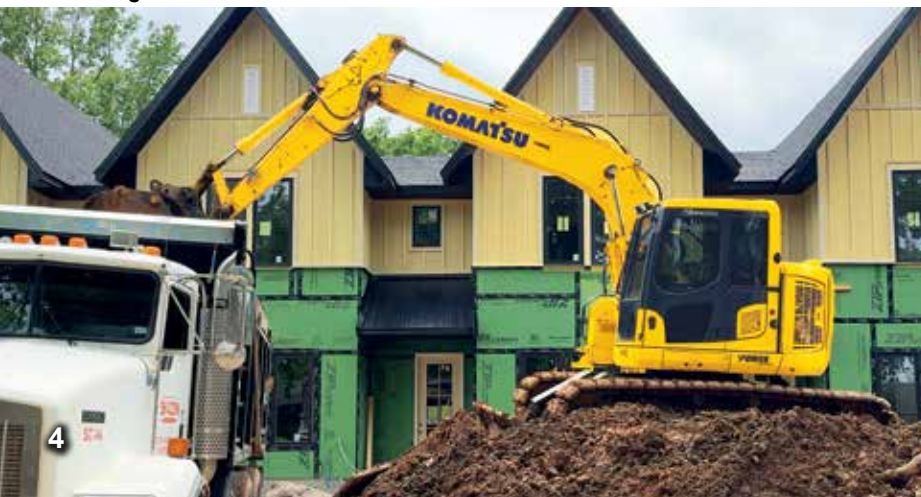
An operator loads a truck with a Komatsu PC138USLC tight tail swing excavator.
