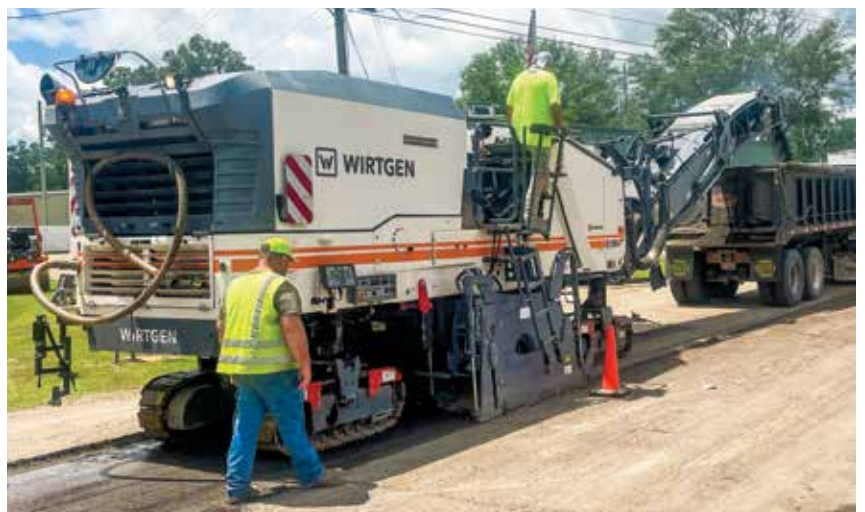
W G Construction mills a road with a WIRTGEN W 200 Fi cold milling machine.
