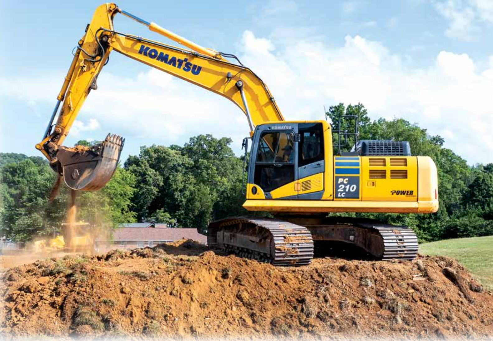
An operator uses a Komatsu PC210LC excavator to pick up material.
